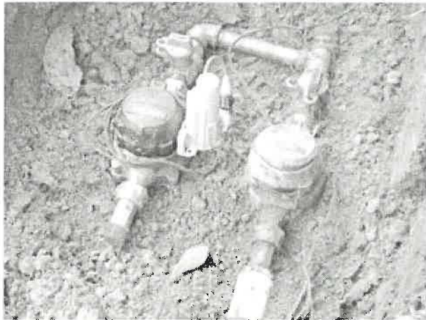
A secondary dedicated irrigation meter is set right next to your existing meter and can significantly reduce your water bill.
