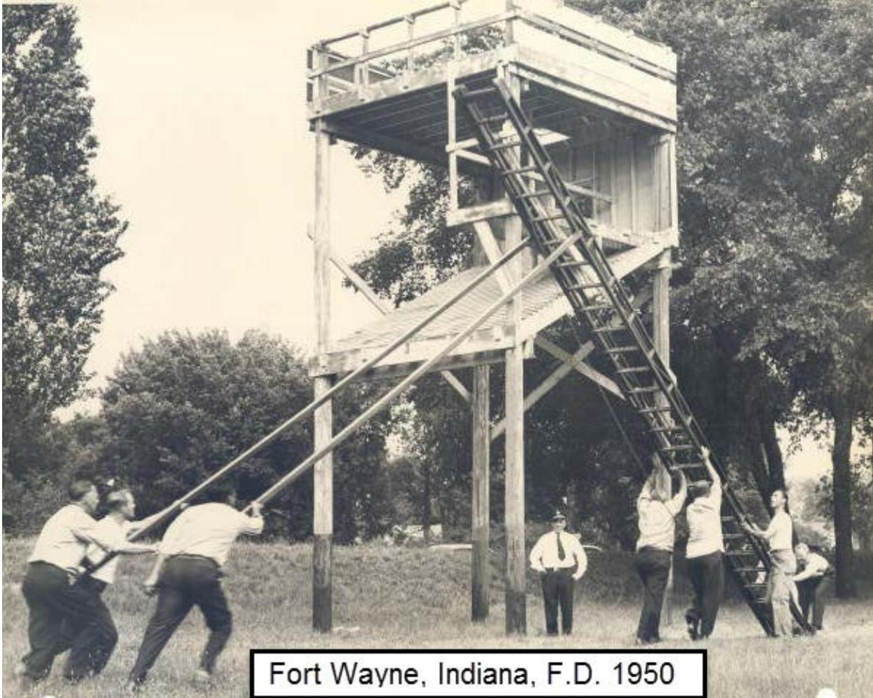
Example of a 3-story wooden drill tower in use. Notice window opening on the rear of the second floor and incorporation of pitched roof simulator.
