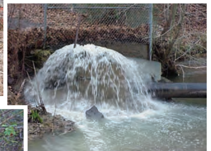
Top: Chronic overflow location prepared for the next event. This overflow has now been corrected. Above: Manhole overflow into a stream.
