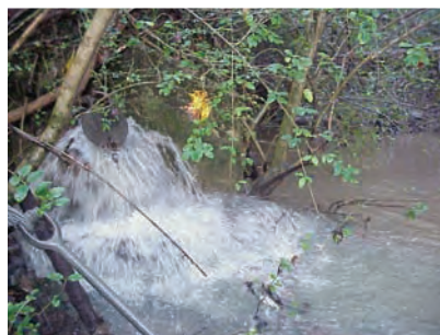
Top: Chronic overflow location prepared for the next event. This overflow has now been corrected. Above: Manhole overflow into a stream.
