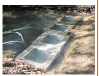
These concrete boxes are part of the stream restoration research project. Shown here, they are approximately 90% installed and will be backfilled shortly for stabilization.
