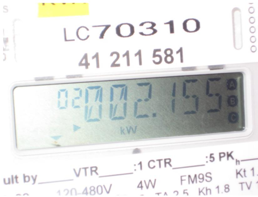
This is a commercial meter showing the kilowatt demand reading. The peak kilowatt demand is  $2.155 * 120 = 258.6$  kW. Demand measurements are returned to zero each month. The readings are in 30 minute blocks of time and represent the peak 30 minute rate of electrical usage during
