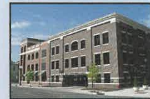
This parking garage in Downtown Franklin, TN, reflects the area's historic architecture. Ground floor retail space would make it even better.
