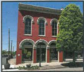
125 Main Ave. - Dragon Fly: painted south & east façades
