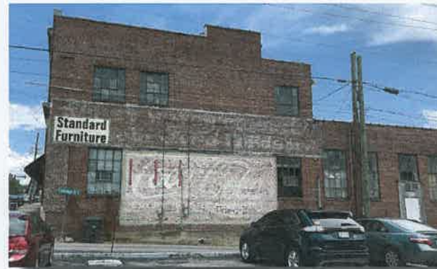
These ghost signs on the south side of a building on the northeast corner of Main and Campbell are prime candidates for a restoration project as described in the sidebar at right.
