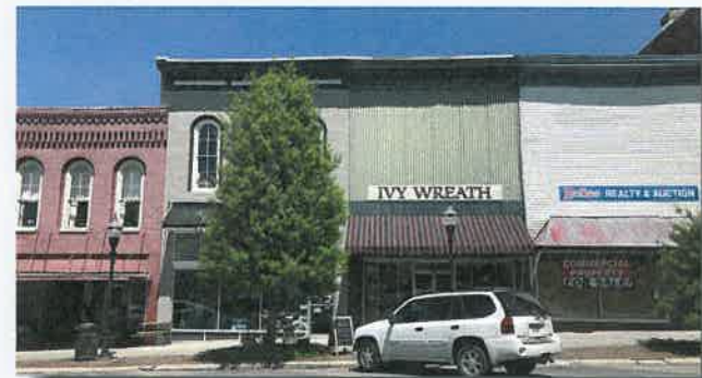
The removal of the mid-20th century “slipcovers” that were applied to the facades of these upper floors would greatly add to Downtown Fayetteville’s overall historic character.
