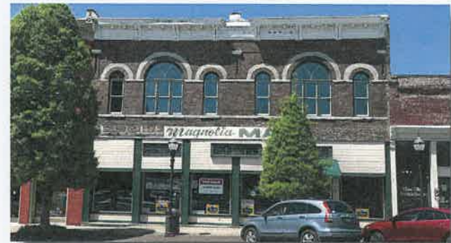
Although the upper floor of this building has been well-preserved, the storefront has been altered and offers an excellent opportunity for a historically-accurate rehabilitation.
