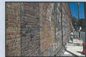
Ghost sign restoration in progress in Mooreville, NC.
