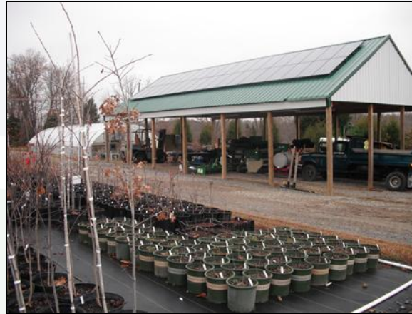
Nashville Natives 8.28 kW system in Fairview, TN
