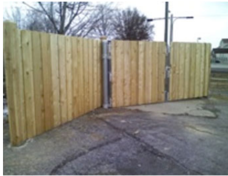
Example: Properly Screened Dumpster
